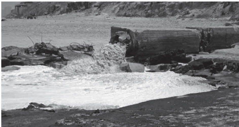
Figure 14: One of many outfalls of untreated sewage into the Mediterranean Sea. 193
