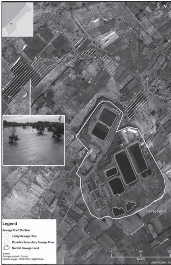
Figure 5: Extent of sewage flood from Al Zaitoun sewage treatment plant as a result of Operation of Cast Lead (Image from 19th January 2009). 4
