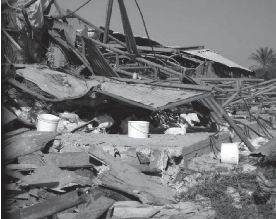
Figure 9: A destroyed poultry farm in Zeitun after Operation Cast Lead. 130
