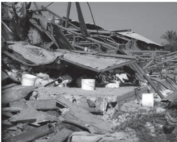
Figure 4: A destroyed poultry farm in Zeitun after Operation Cast Lead. 3
